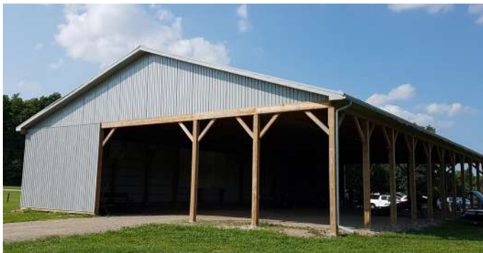
Figure 10: Photo of Existing Pavilion (2021)
