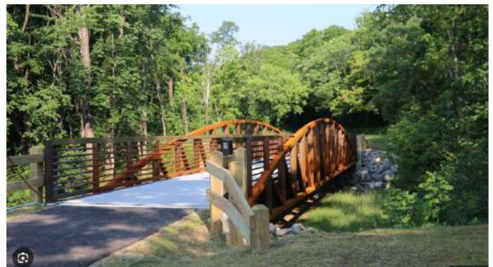
Figure 23: Drainage feature with bridge. Source: The Roanoke Star News
