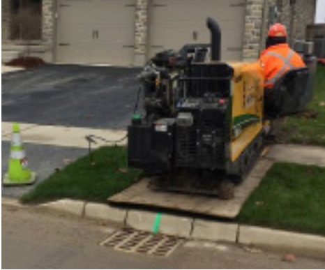
Drop install Small directional drill
